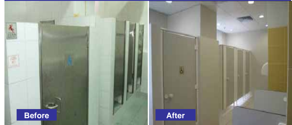
Waldorf: Upgrading of washroom
