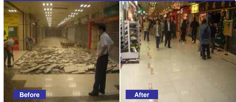
Waldorf: New floor tiles in main corridor
